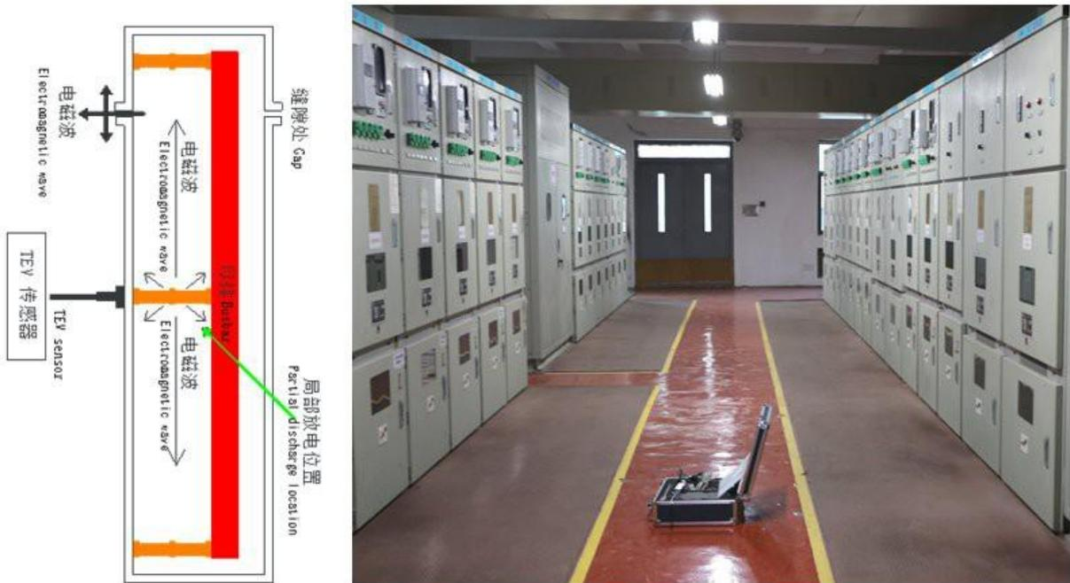
Figure 3-1- TEV detection schematic
